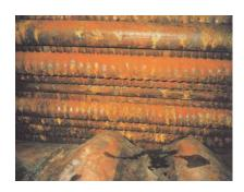
In addition, the corrosion sediments create a bed for bacteria that feed off of the corrosion. These bacteria, found under the sediments, feed off the iron dissolved by the acids that the bacteria produces. The most common solution, adding chemicals, doesn't adequately solve the problem and causes damage to pipes, accessories and auxiliary equipment.
